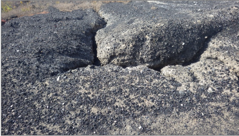
Photo 13, Point 13 Boiler Slag Pond – Southwest Divider Dike – Erosion gully at the crest.
