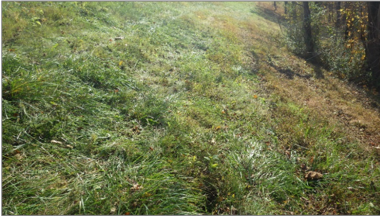
Photo 16, Point 16 Boiler Slag Pond – West Exterior Slope – Erosion gully near the crest.
