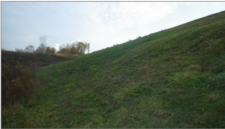
Photo 32, Point 31 Northwest Exterior Slope – Bare spot on the slope near mid- height.
